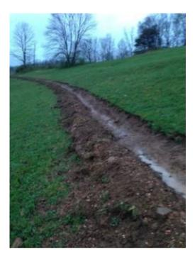
New grassed shallow ditches are required to be constructed by the 1st October 2022. This gives time for seed to establish before winter and provides more effective runoff attenuation.
